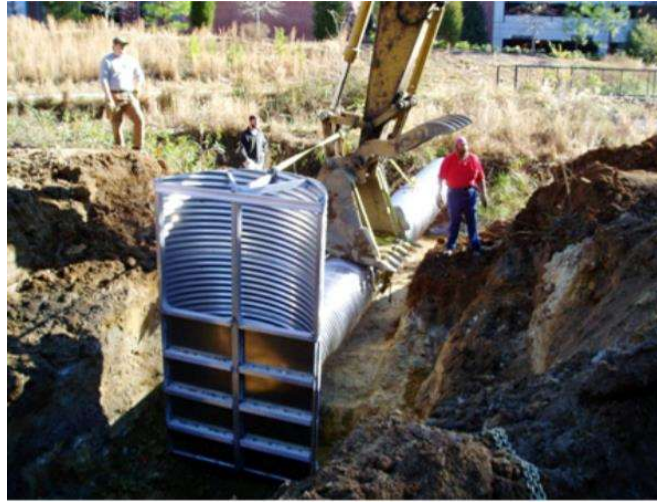
Figure 12. An example of a flashboard-controlled outlet (flashboard not pictured). Water outlet elevation can be controlled via a drain pipe constructed through a berm (NC State 2020).
